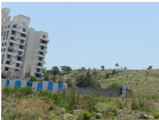
Construction on Hill slope (Bavdhan Area)
