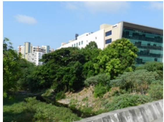
Construction and Dumping near channel
