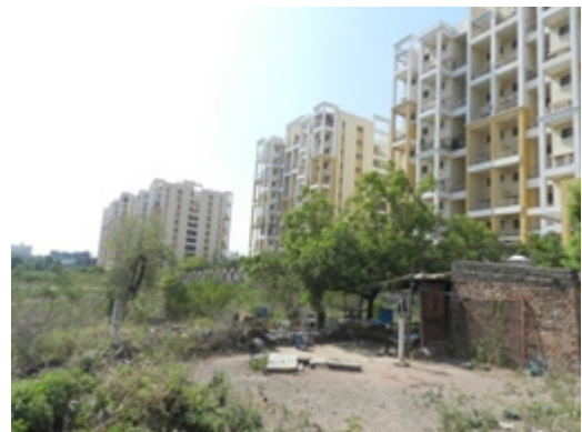
Construction on Stream (Banner - Pashan Road)
